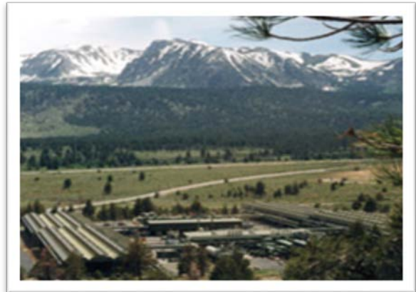
Geothermal Power Plant Inyo National Forest, California
